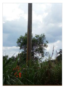
A base offset should be used for collecting IKE Photos of poles where the base of the pole is not visible due to vegetation, snow, or anything that obscures the base.
